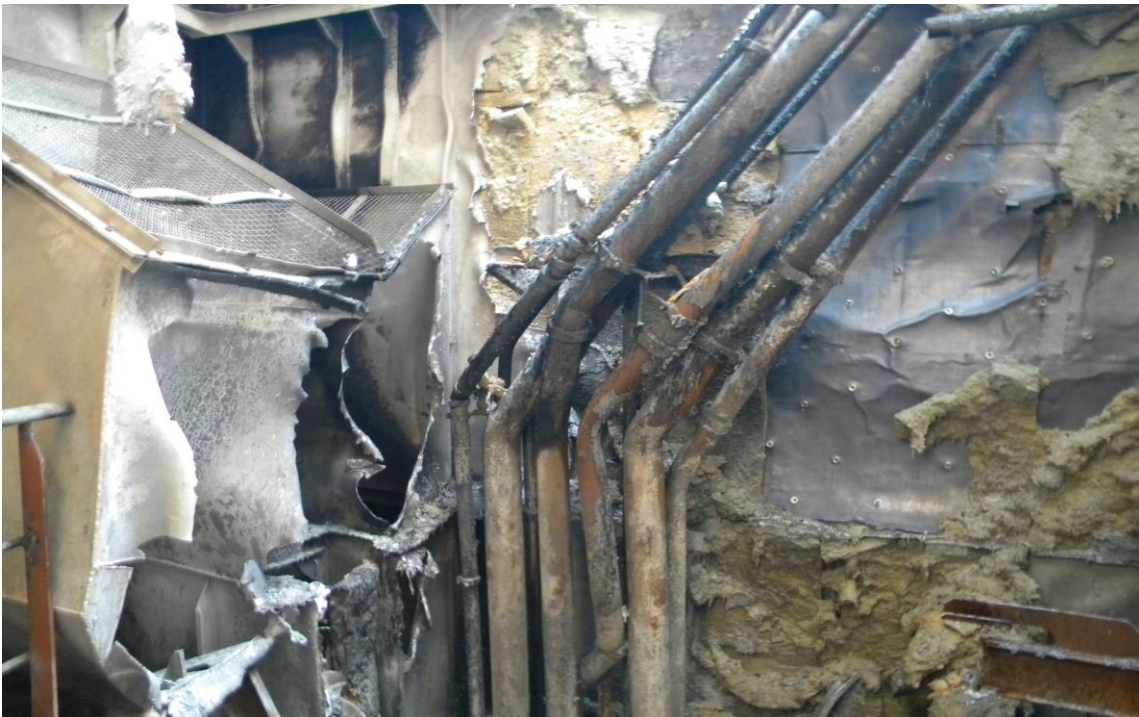
Figure 20: Deck 14 ducting for generator air supply, bioreactor exhaust fan, scupper drains, exhaust gas boiler safety valves, air conditioning system drains and pre-heating cooling system drains
