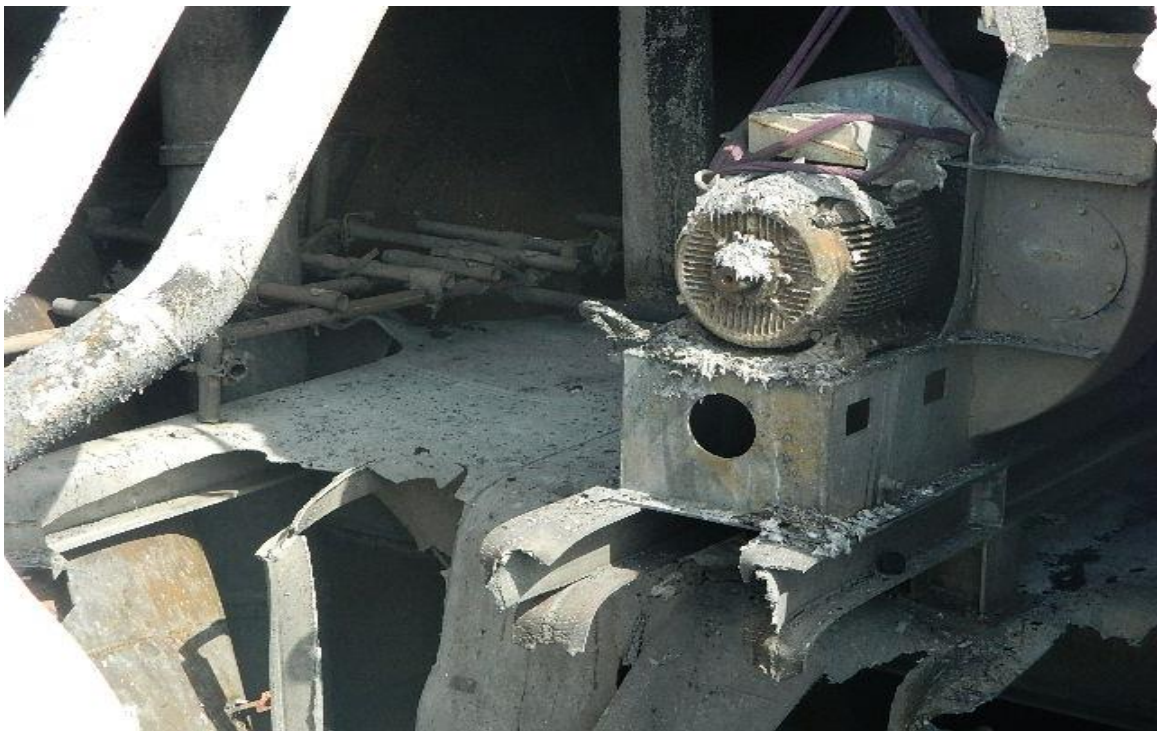
Figure 18: Deck 16 air sealing fan installation, recently installed but not commissioned
