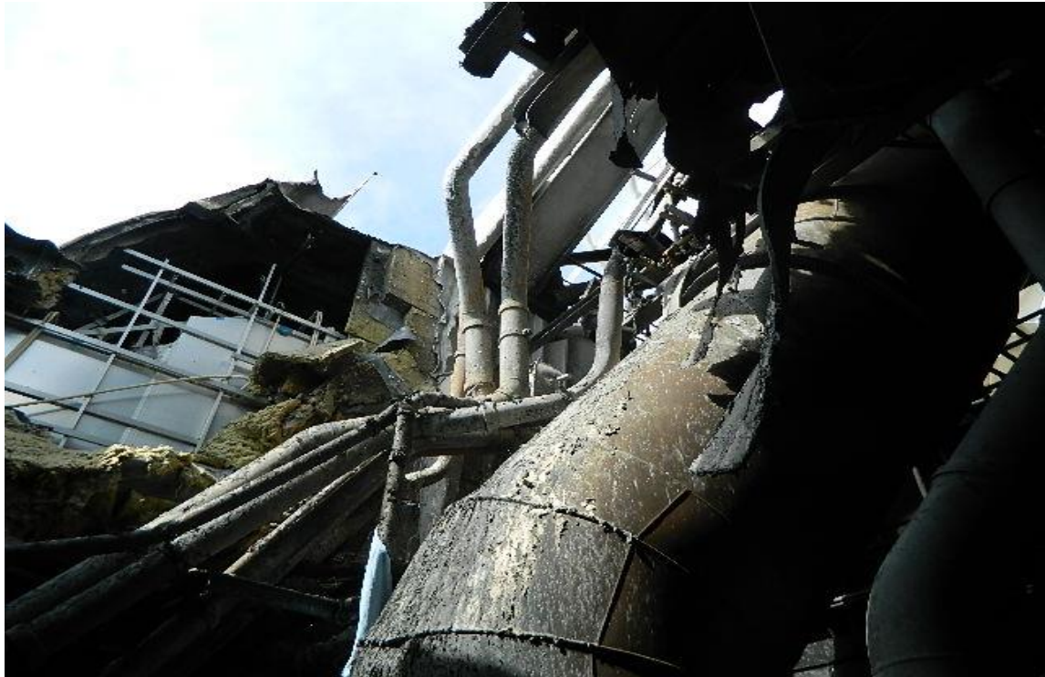
Figure 17: Internal damage at Viking Crown, deck 16. Exhaust duct from generator No.3, pre-heating cooling system, scupper drain lines, exhaust gas line from boilers, safety valves and air conditioning drain lines damaged
