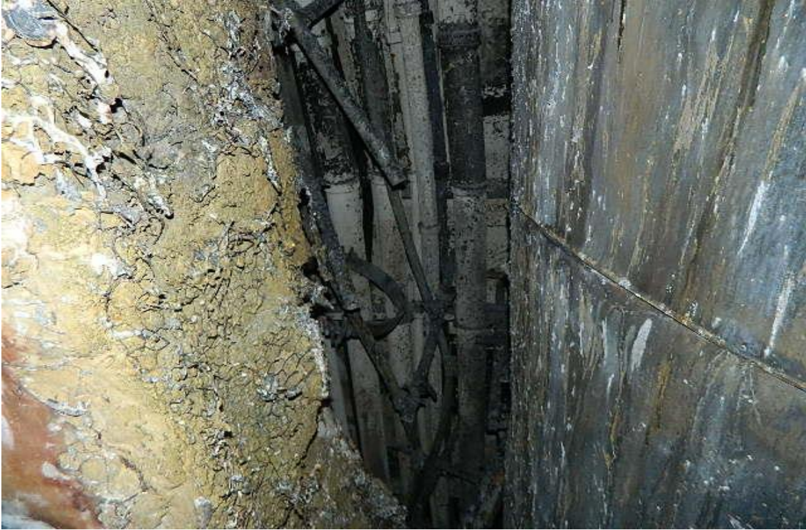
Figure 23: Deck 8, insulation and coating damages
