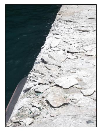
Figure 19: Damages to the quay
