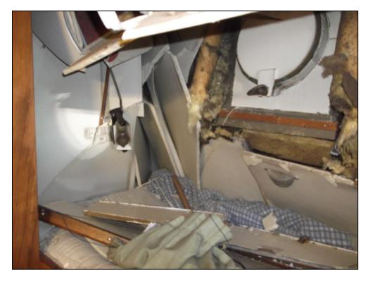
Figure 21: Internal damages on *Union* (chief mate's cabin)
