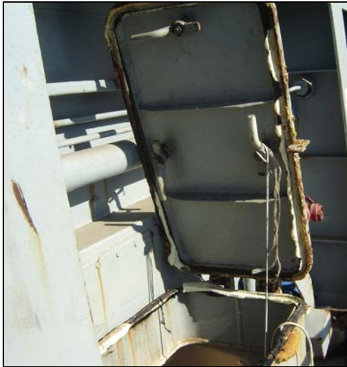
Figure 1: Starboard cargo hold access shaft from the main deck
