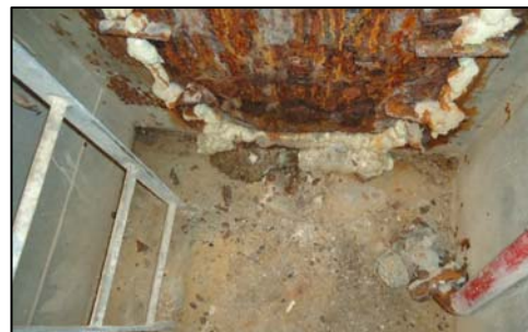
Figure 5: Access hole leading to the cargo hold sealed with expanding foam
