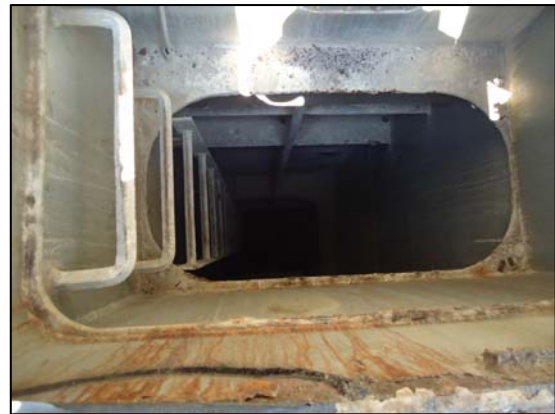
Figure 2: Starboard cargo hold access ladder from the main deck
