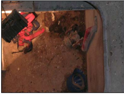
Figure 8: Condition of the access shaft several hours after the accident
