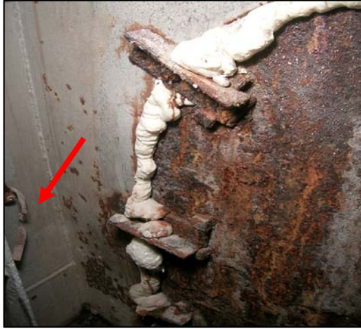
Figure 12: Portable fire extinguisher strap located in the access shaft where the accident happened
